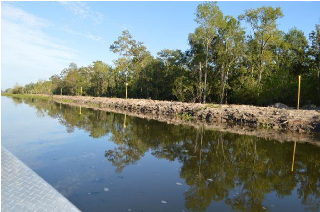
Fig. 1-W. September 11, 2019. This photo depicts Bayou Bridge pipeline markers in the spoil bank, and an absence of gaps in the spoil bank. Dean took this photo facing northeast, traveling northwest in the canal adjoining the right-of-way between the dike northwest of Bayou Chene
