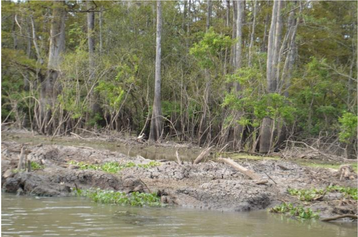
Fig. 2-E. This photo depicts illegal fill/Clean Water Act violations along the pipeline right-of-way after construction, and dirt in the adjoining forest likely as a result of digging during high water without using appropriate, required erosion controls. Dean took this photo facing north, with the pipeline trench in the bottom portion of the photo, between the following approximate coordinates: 30° 05'24.32" N, 91° 21'10.19" W to 30° 05'10.71" N, 91° 23'51.29" W.
