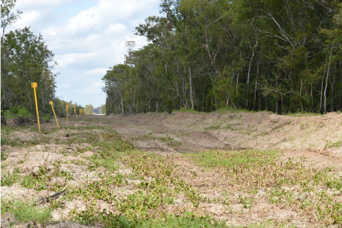
Fig. 3-W. September 27, 2019. This photo depicts the extent of the illegal fill/Clean Water Act violation along the pipeline right-of-way. The pipeline is on the lower part of the picture without markings. The picture was taken facing northeast, approximate coordinates: 30° 07'38.37" N, 91° 34'27.79" W.
