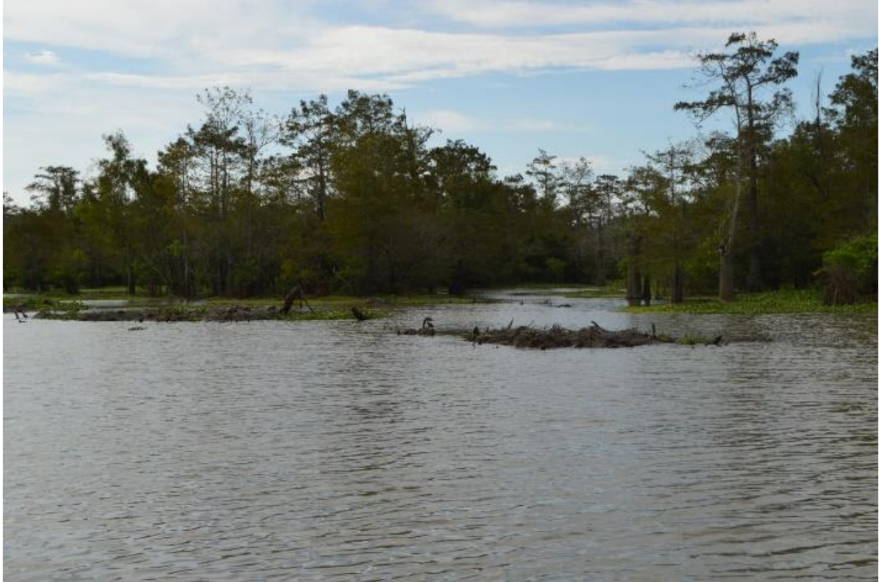
Fig. 8-E. This photo depicts another pre-existing, unnamed slough, that is dammed by debris, another illegal fill/Clean Water Act violation. Dean took this facing north, at a location west of Cross bayou between the following approximate coordinates: 30° 05'12.84" N, 91° 22'38.47" W and 30° 05'10.71" N, 91° 23'51.29" W.
