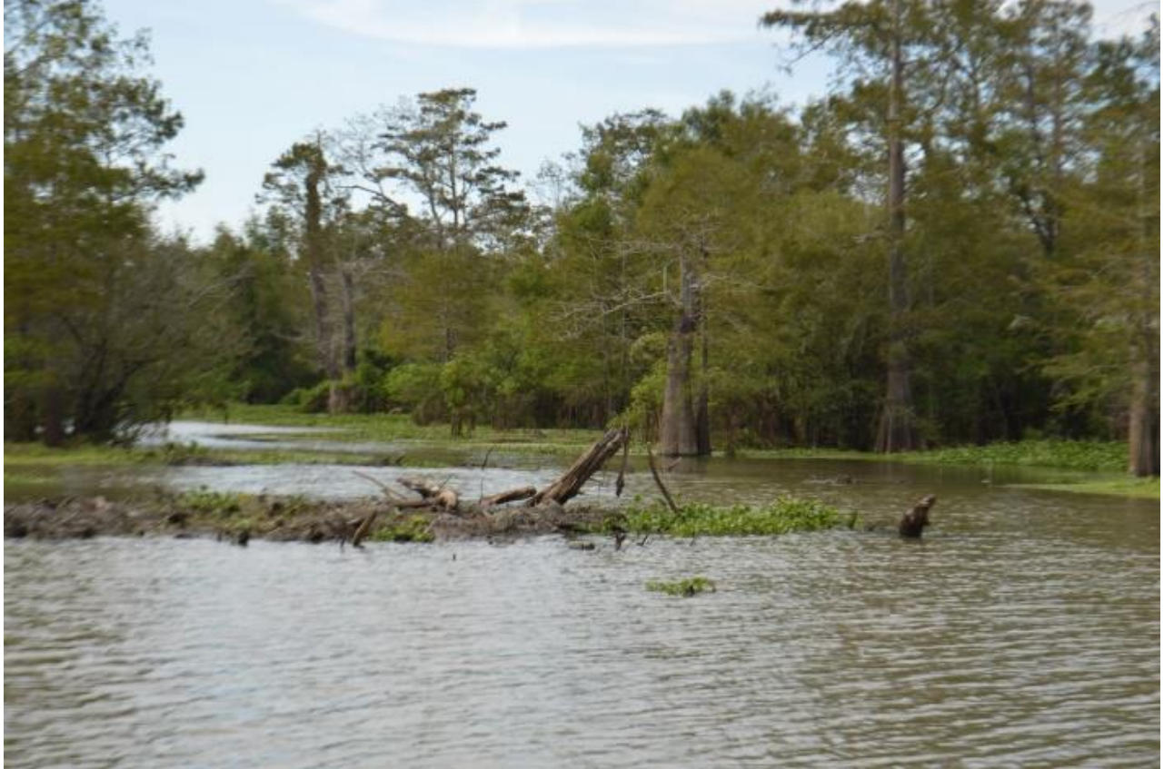
Fig. 7-E. This photo depicts another preexisting, unnamed slough, that is dammed by debris, another illegal fill/Clean Water Act violation. Dean took this facing north, at a location west of Cross Bayou between the following approximate coordinates: 30° 05'12.84" N, 91° 22'38.47" W and 30° 05'10.71" N, 91° 23'51.29" W.
